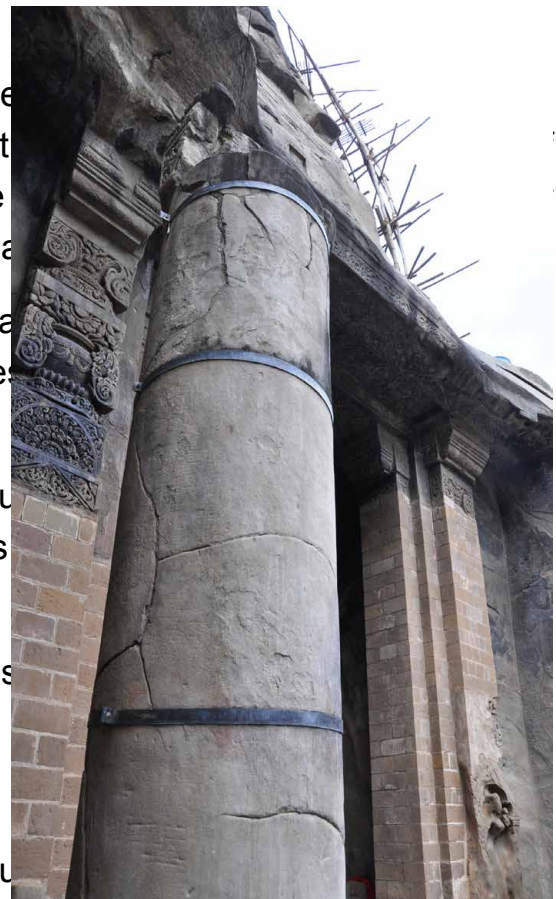
fig. 29 Columns of mandapa
