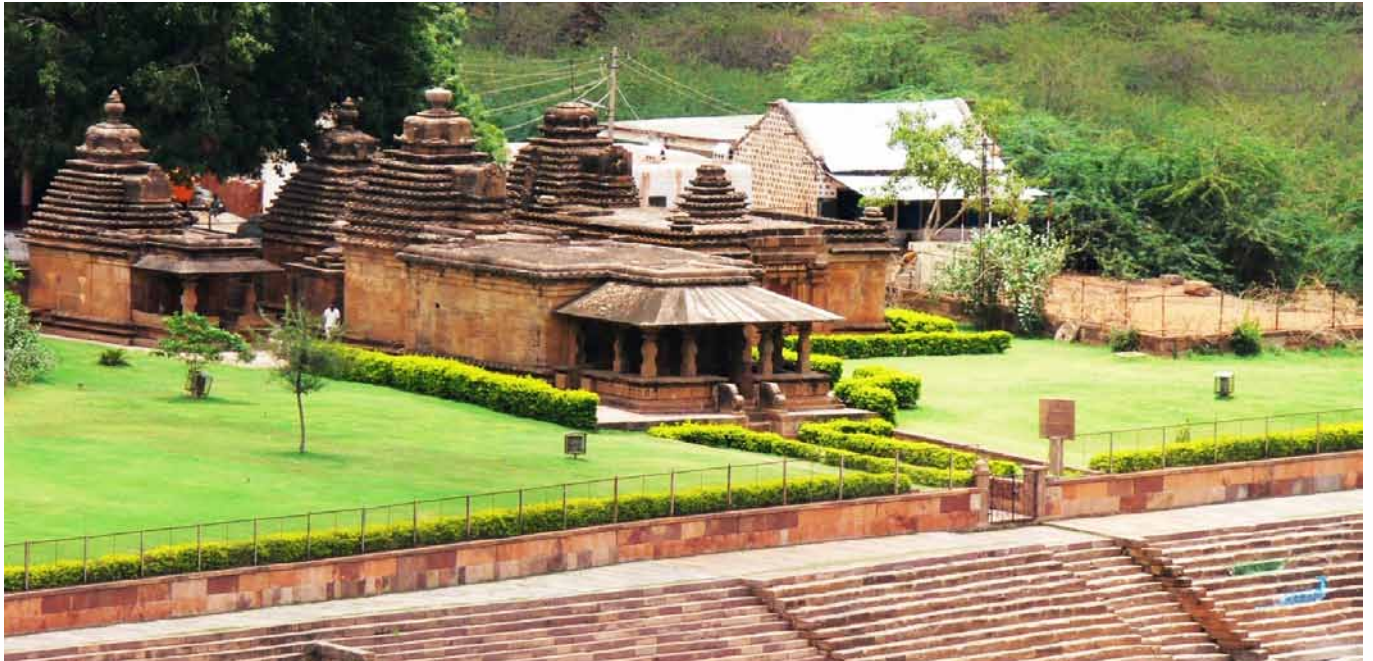
fig. 63. North Bhootnath Group of Temples: These temples belonging to the 11th-12th century CE have peculiar layered pyramidal towers, closed mandapas, plain outer walls and pillared half open porches with balcony seating.
