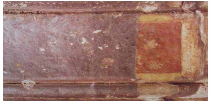
fig. 28. Cave no. 17, Ajanta: Removal of soot from pilaster
