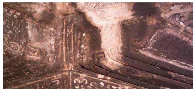
fig. 29. Ajanta: Pillar brackets infested with bat excreta
