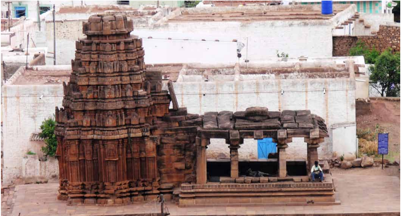
fig. 65. Yellama Temple: Originally dedicated to Lord Vishnu, this late Chalukyan (12th century CE) temple has an experimental combination of elements of both the Nagara and Dravidian architectural styles interestingly displayed in its sikhara along with the peculiar inner lathe-turned pillars of the mandapa.
