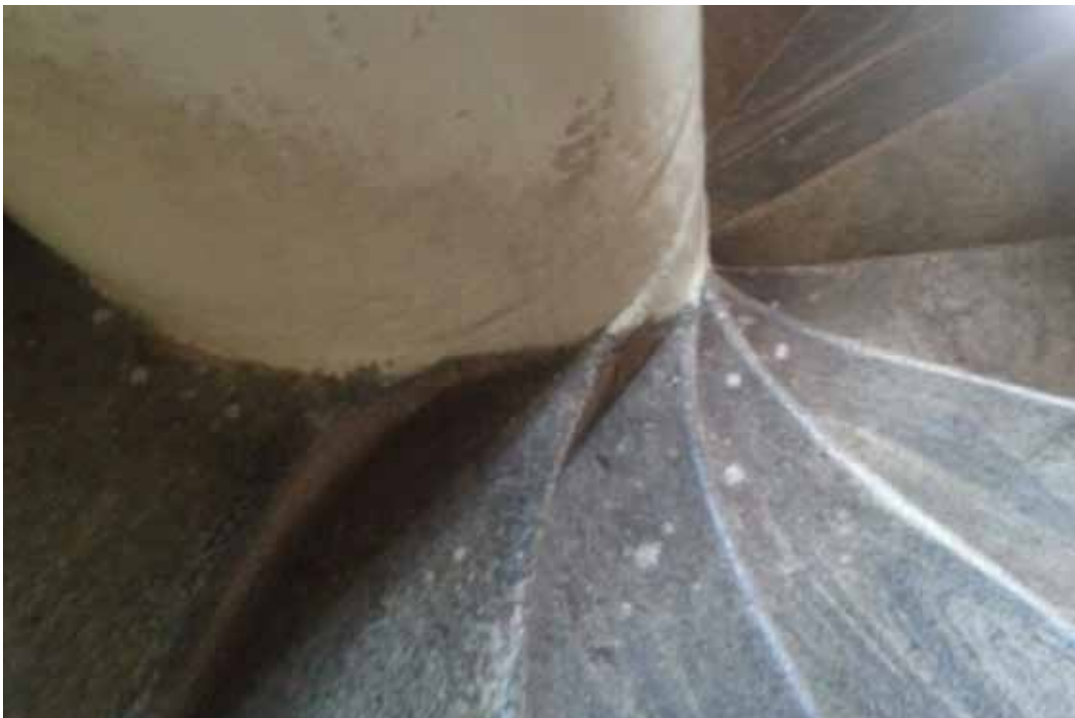
fig. 38 Indigenous materials like granite used as flooring in the museum: Archaeological Museum, Bangalore
