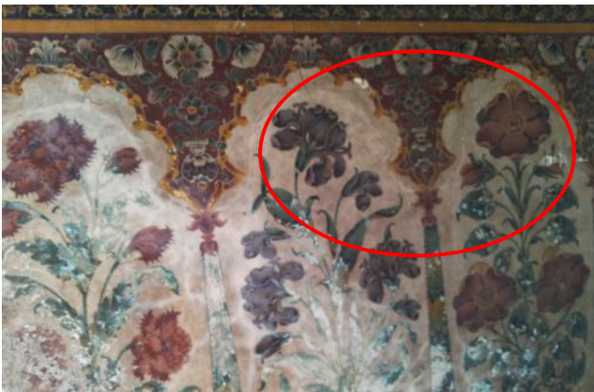
fig. 1 Golden Temple, Amritsar: Stains over paintings due to disruption in dispersal of moisture from inside
