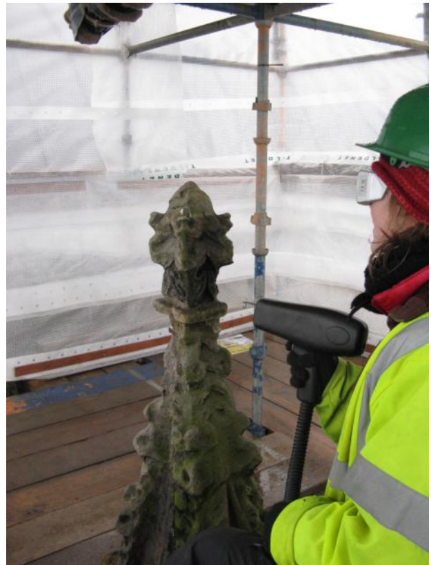
fig. 1 Use of laser cleaning machine for the removal of pollutants (Source: Gurpreet Singh, 2011)
