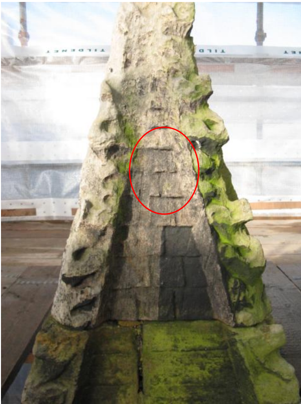
fig. 2 Cleaned sandstone surface by using laser cleaning machine (as marked in red circle) (Source: Gurpreet Singh, 2011)
