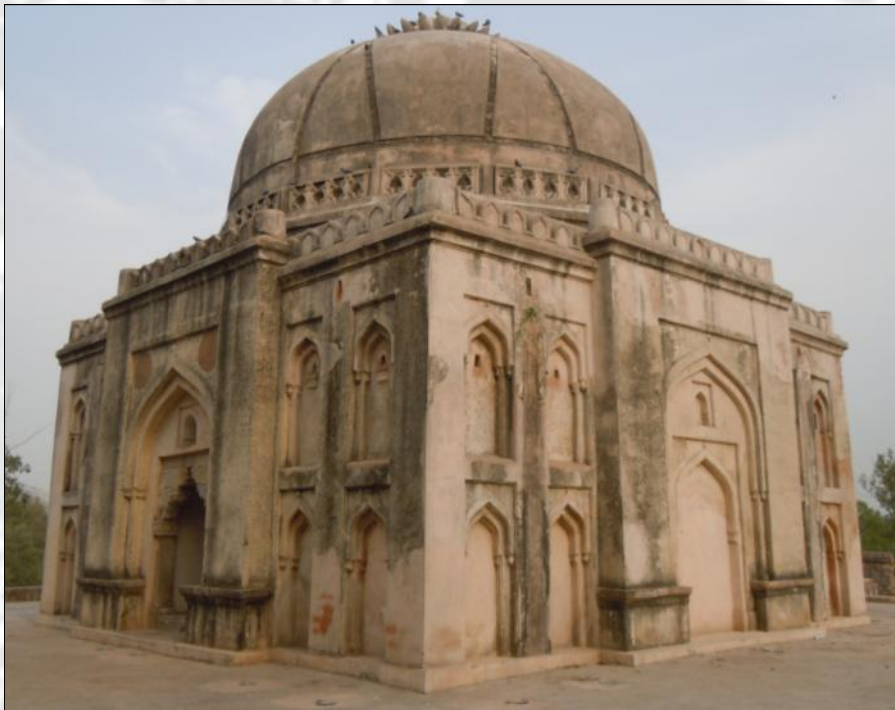
fig. 8: Bara Lao ka Gumbad (after completion)
