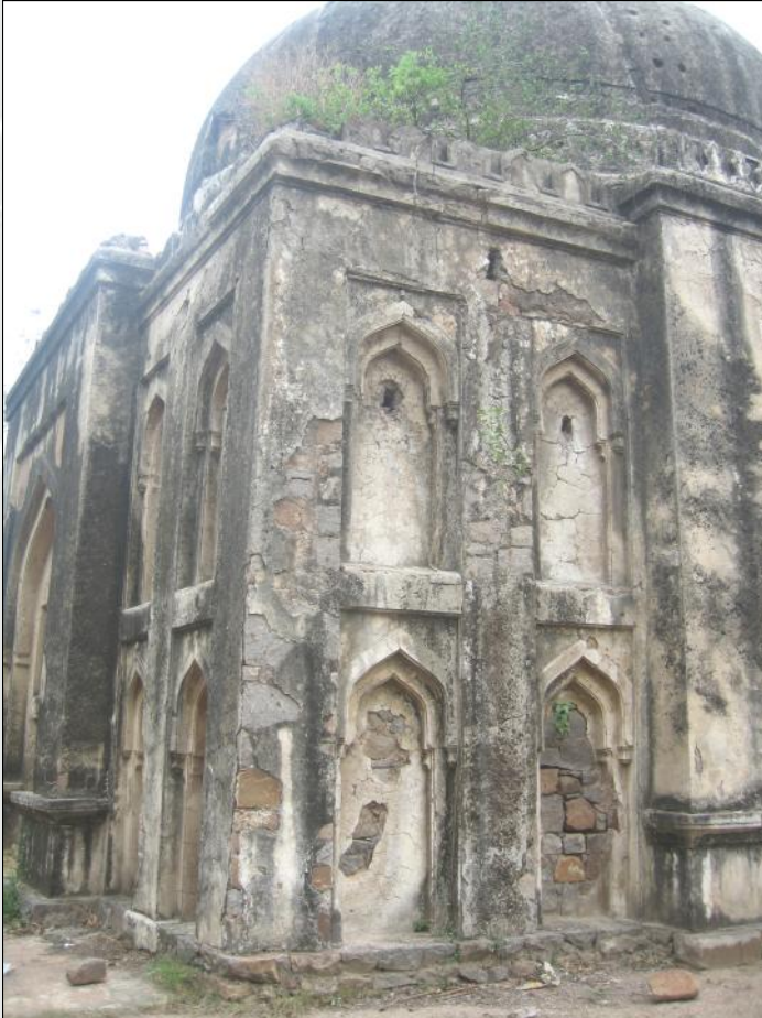
fig. 3: Damaged plaster
